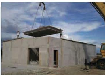
Through a mutual relationship, CON/STEEL Alliance™ member STAR Inc. of Amherst, Ohio, partnered with Double Harvest to build a tilt-up concrete cooler. The 2,400-square-foot cooler features insulated concrete roof and wall panels to create the optimal thermal envelope. The cooler has a center dividing wall so farmers can control their energy consumption when only one side is being used.
